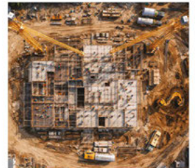
CONSTRUCTION & DEVELOPMENT Monitor construction progress
