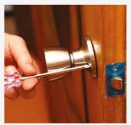
setback stamped on them, but if not, use the tape measure or a ruler to measure from the edge of the door to the center of the hole. Standard doorknobs will have a backset of either 2 3/4 or 2 3/8 inches. If you have any question about the backset, just carry the old latch with you to the hardware store.
