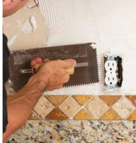
The natural stone of travertine has much variation, so laying them out in advance helps you avoid any surprises while placing them in mortar. After mocking up your pattern, measure a block of your design and mark those dimensions along the wall where they will
