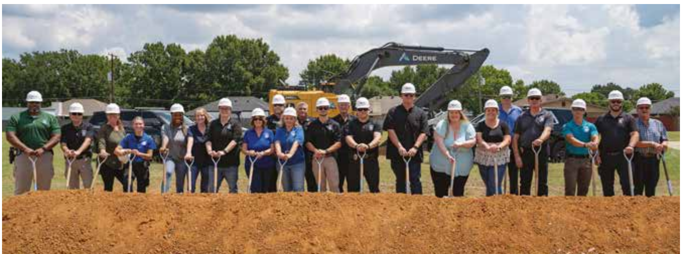
The city of Burlison breaks ground for the Burlison Police Department Headquarters Expansion.
