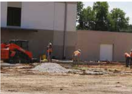
Construction crews work diligently to finish the new location for Center of Hope.
